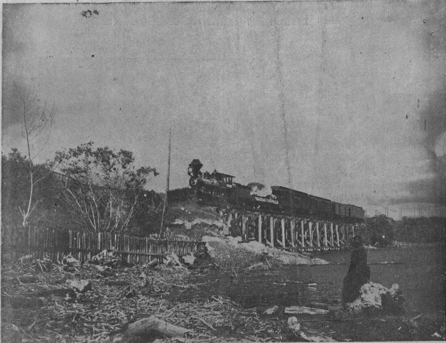
The old railroad trestle at Wood's lagoon was new when this unidentified woman sat on
