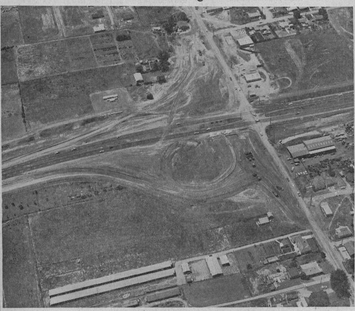
From the air, the area around 41st avenue looks as if some giant hot-rod had churned up the soil in great sweeping, skidding circles. But in reality all this area is needed in the construction of the 41st avenue over-crossing. Fifty-five thousand tons of dirt is being used to build the ramps leading up to the overcrossing. Said to be 30 per cent completed the labor and material cost for the crossing is about \$530,000.
