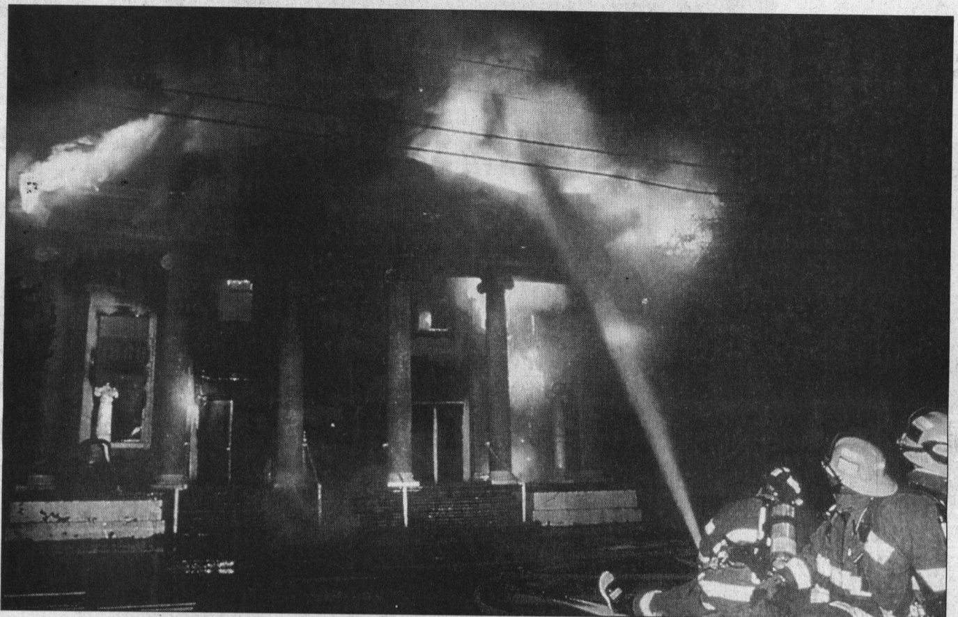
Santa Cruz firefighters battle the blaze at Grace United Methodist Church in October 2000. Shmuel Thaler/Sentinel file
