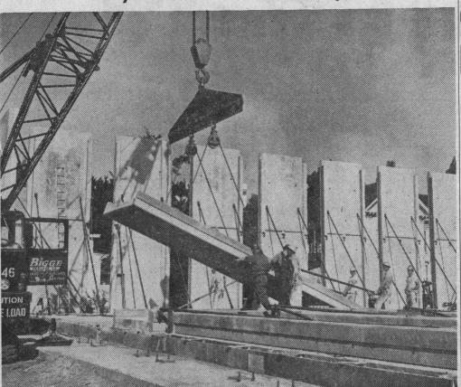
A mammoth crane today is lifting the 15-ton pre-cast wall sections of the city hall addition into place. The \$400,000
