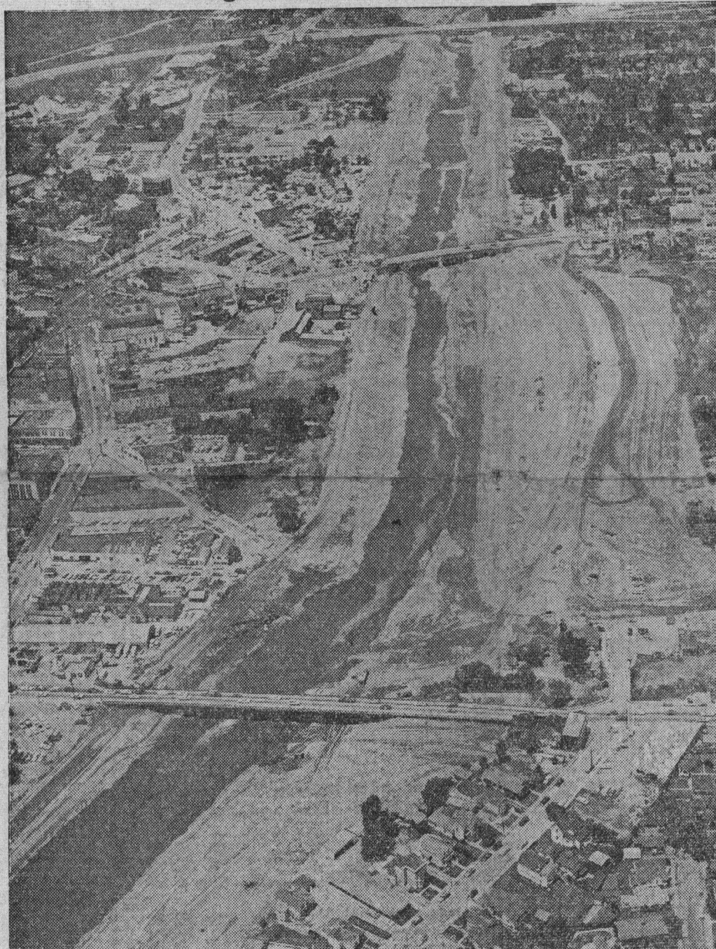
The above aerial photo shows the Granite construction company line of march from the business district by-pass bridge (top) to the Soquel avenue bridge. Granite officials said last week that levee forming and shaping between the two points is nearly complete. Later work will include sprigging with ice plant and studding with riprap.
