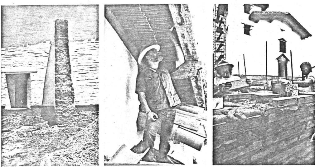
*Proof of Sanchez's commitment to authenticity abounds: A buttress on the south side of the chapel is left exposed so visitors can see the adobe; rawhide ties, which Sanchez is shown checking under the bell tower, are used to attach thatching to hand-hewn beams; and an adobe wall, like one that surrounded the original mission, is being built in front of the chapel.*
