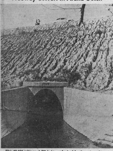
This 90,000-cubic-yard fill is in Arana gulch along the new free-way. It is 500 yards long and the earth was taken from cuts. Arana gulch creek runs through the 10-foot culvert. Its size is em-
