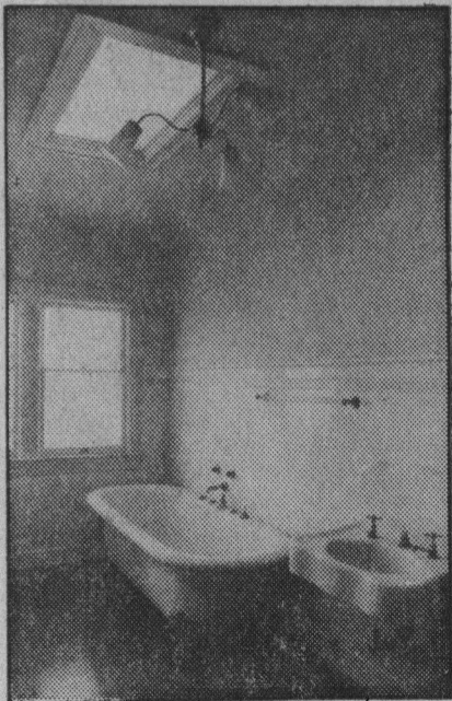
Original tile, fixtures in Goodfellow home.
