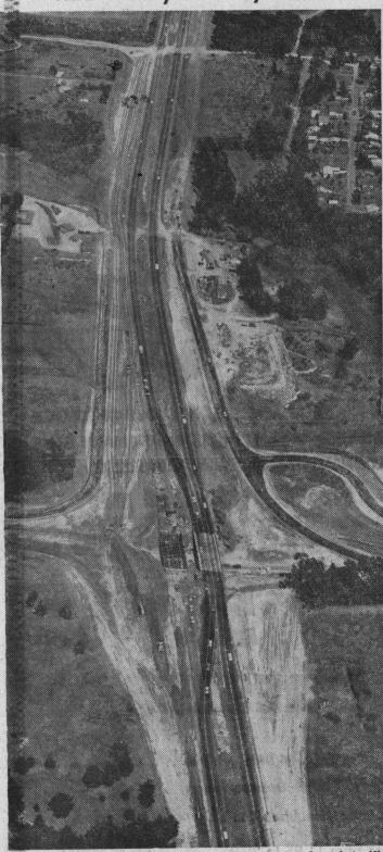
This aerial photo shows detours and frontage road work on the Santa Cruz-Watsonville freeway at Park avenue, Capitola. Santa Cruz-bound traffic must switch over to the recently completed bridge to permit crews to build the parallel structure. sho
