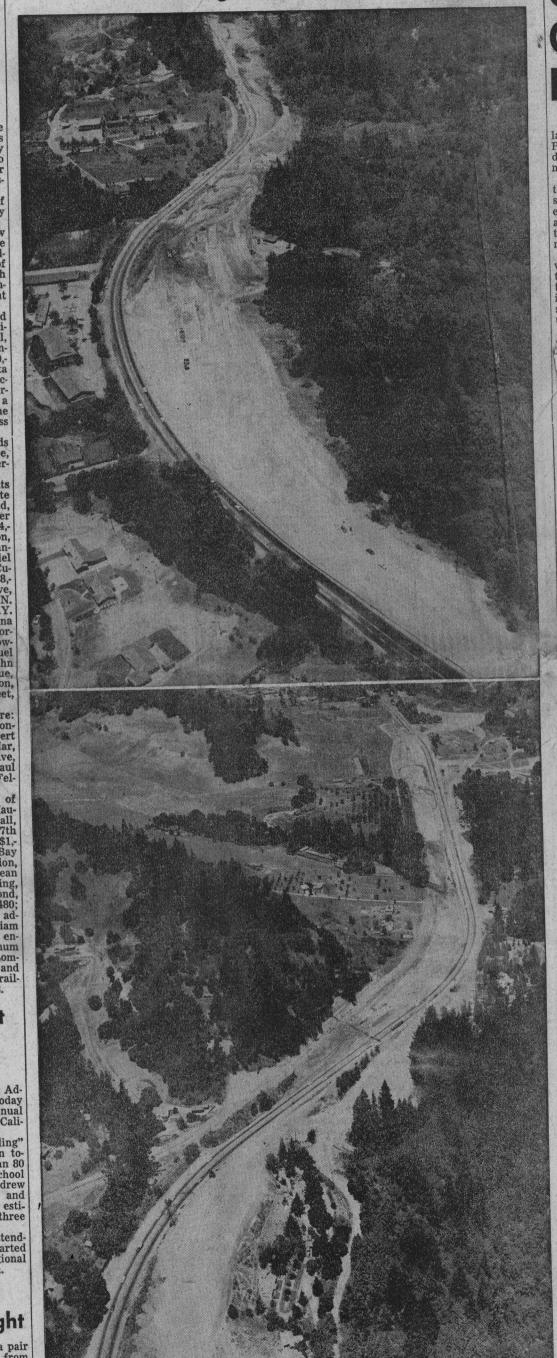
Powerful dozers and scrapers are cutting a huge swath along either side of Highway 17 in preparation for the construction of four lanes of divided highway. The aerial photos above
