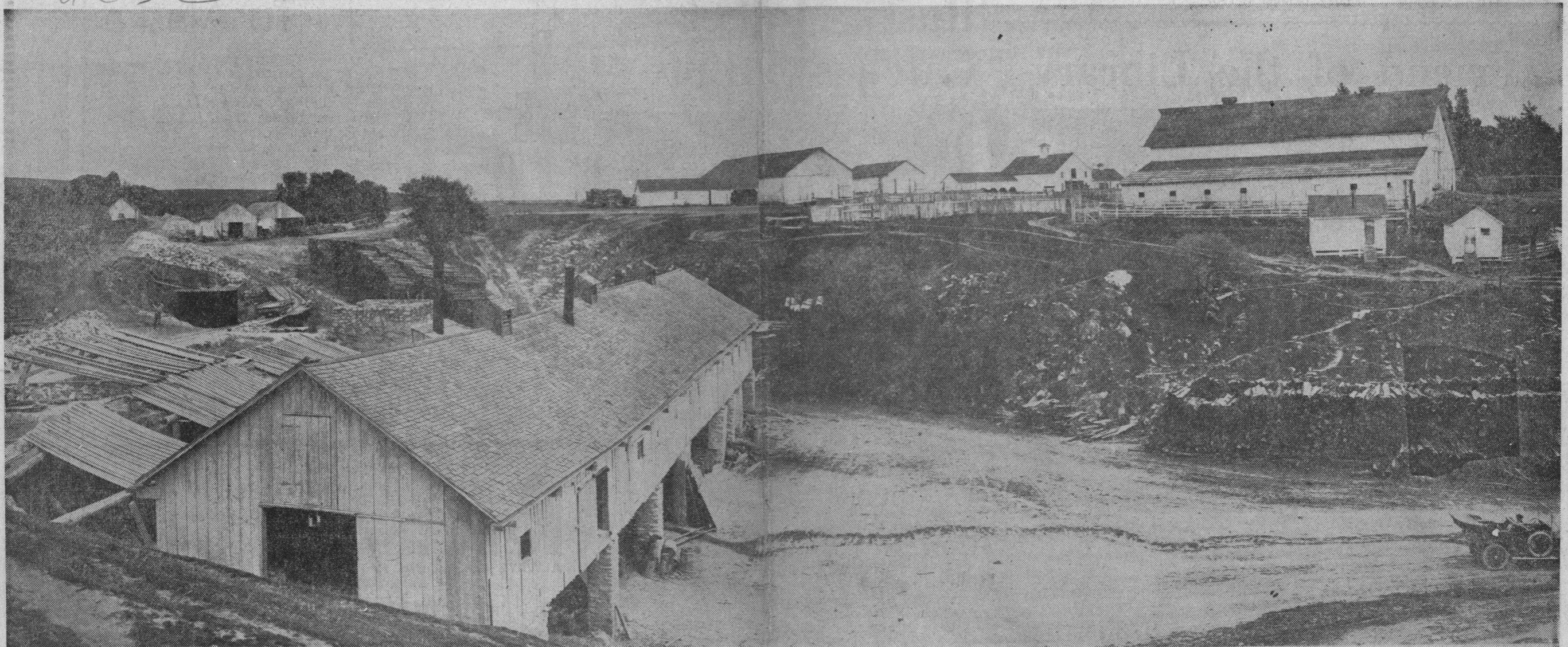
This Cowell Ranch panorama was probably snapped about 1910. The Ranch had recently switched from wood to oil fuel (note new black oil tank on hill at left) for its lime burning operation. The changeover was made in 1908. Still standing are the cooperage (left fore-
