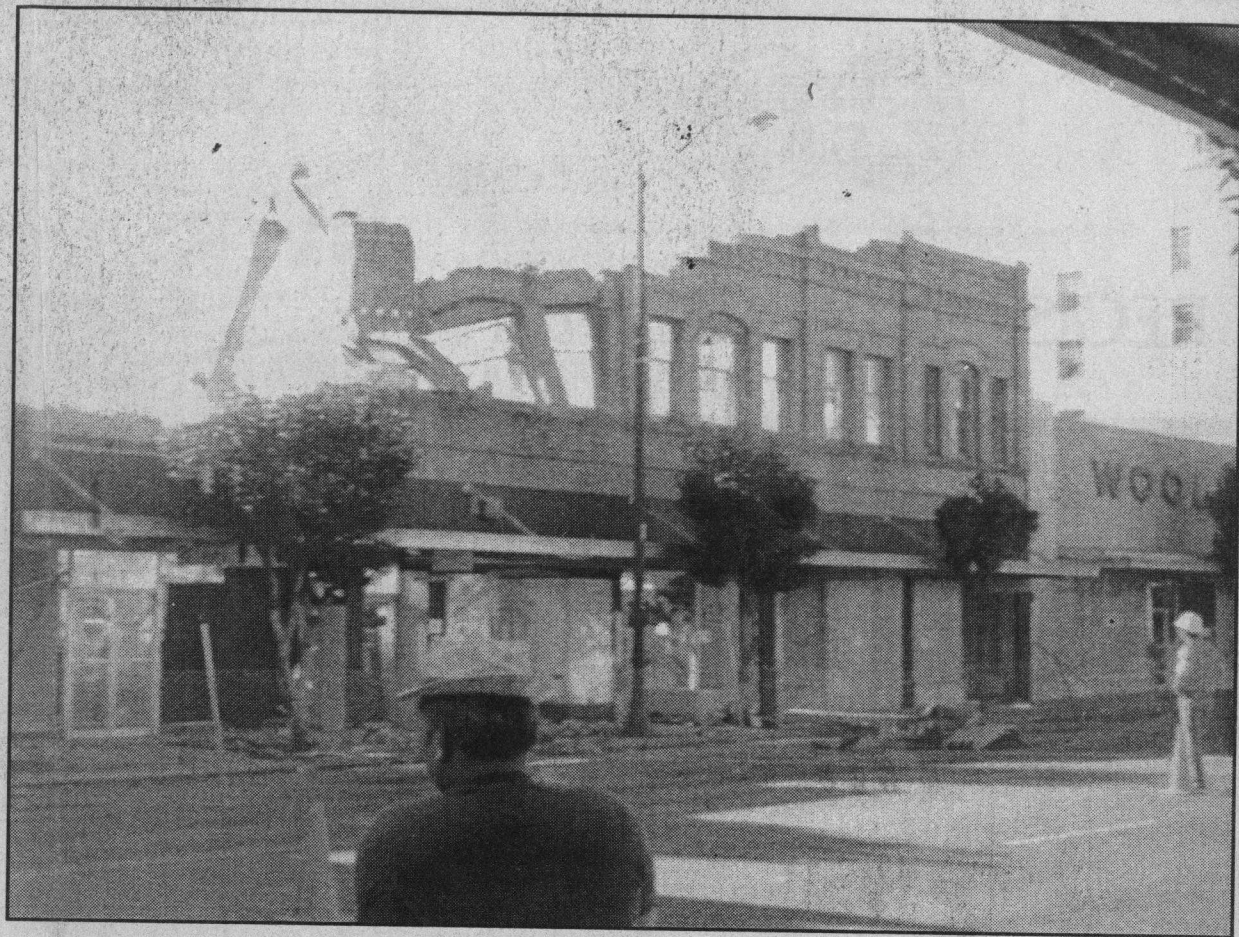
The 400 block of Main Street after the Loma Prieta earthquake in October of 1989.
