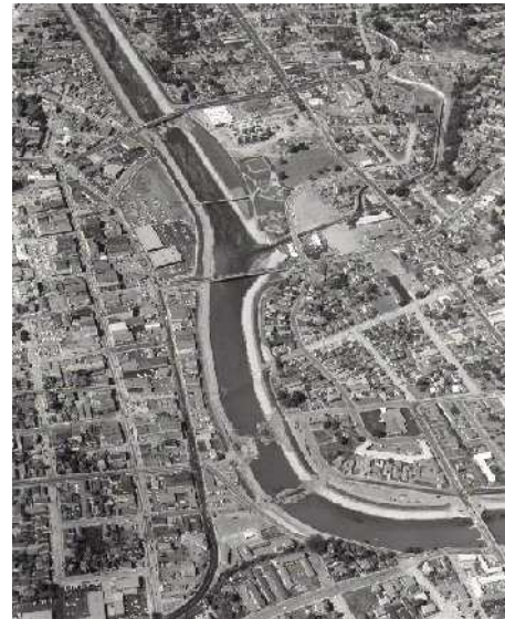
San Lorenzo River Flood Control Project, circa 1967 - Photo by Ed Webber, Provided Courtesy of Daniel McMahon
