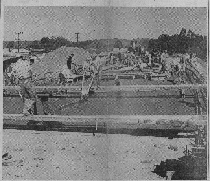
Workmen busily pour and finish concrete decking on the northerly half of the 41st avenue overpass of the Watsonville-Santa Cruz freeway. This phase of the \$527,000 41st avenue interchange project is slated for opening by December 1, according to Gerald Sommers, assistant state highway engineer.
