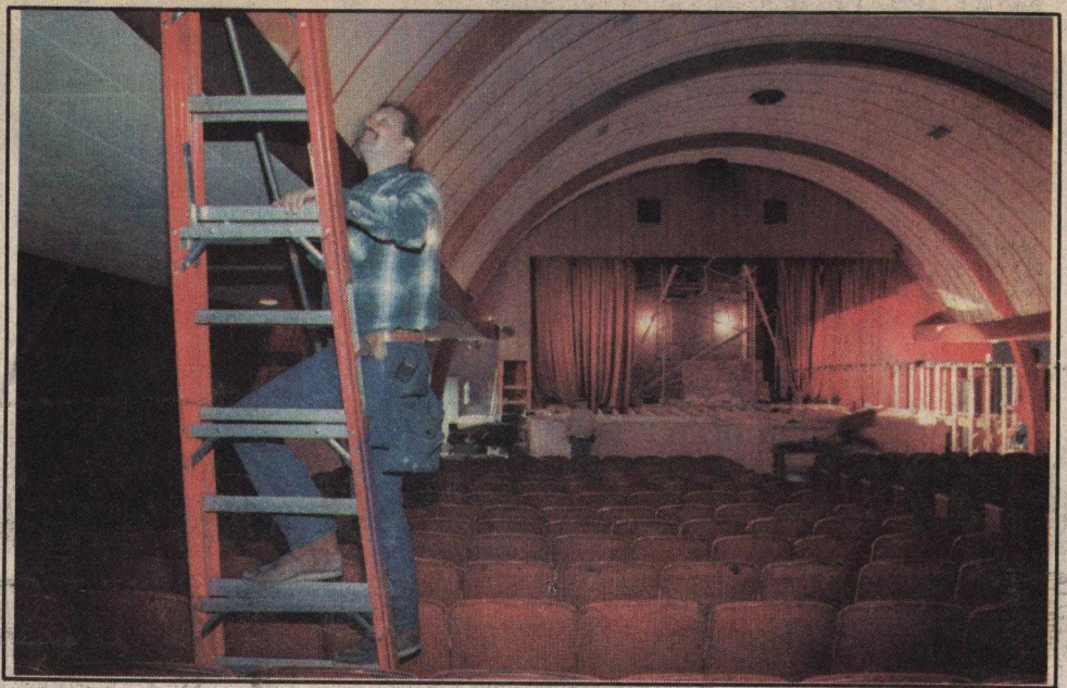
Electrician Pierre Andre helps get the Capitola Theater ready. Shmuel Thaler/Sentinel
