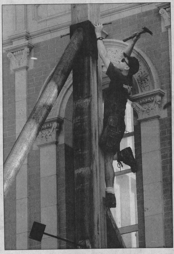
David Martin knocks a pin from one of the steel braces, above, that have been helping to support the walls of the 1894 County Bank building, right, on Pacific Garden Mall in Santa Cruz. Badly damaged in the 1989 Loma Prieta earthquake, the building has been gutted and a new two-story structure is being erected behind the Renaissance Revival-style walls. The five first-floor retail businesses and second-floor offices are expected to be ready in February.
