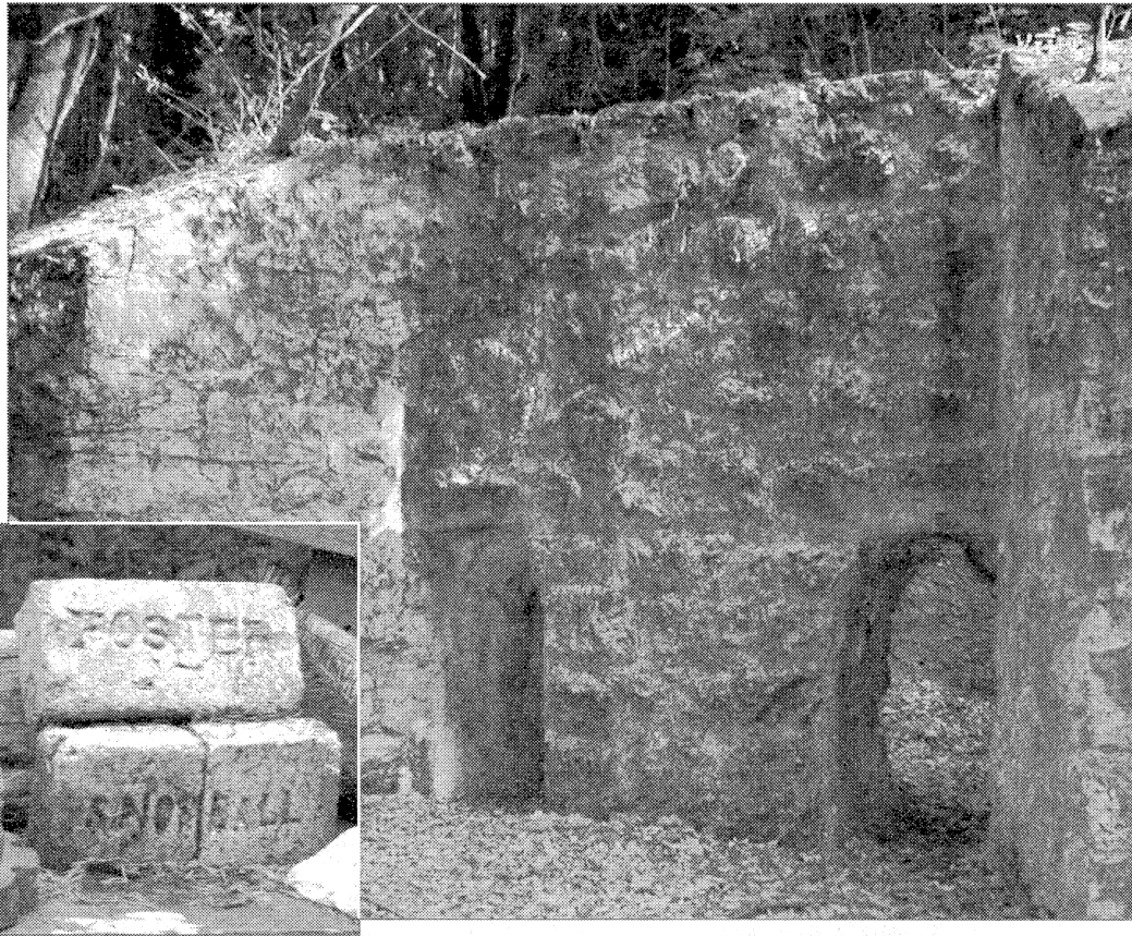
Remnants of a lime kiln in the Santa Cruz Mountains, and (inset) two bricks from "Brick Bat Bob's" collection. Snowball was an English brick manufacturing company of the 19th and early 20th centuries.
