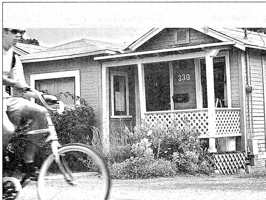
A 1906 earthquake cabin on 9th Avenue in Live Oak.
