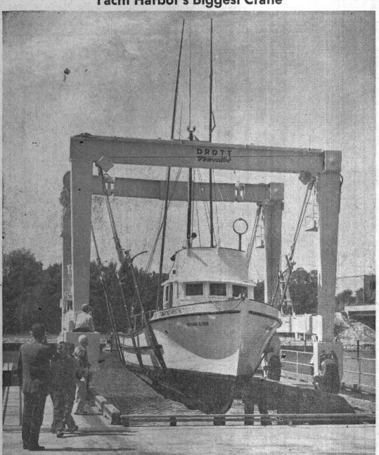
The biggest crane in the Santa Cruz harbor is this "Travelift," part of the equipment at Harbor Marine. The lift, which can handle boats up to 55 feet and 36 tons, has drawn sizable crowds of sidewalk superintendents recently. The boat seen in its clutches, above, is a
