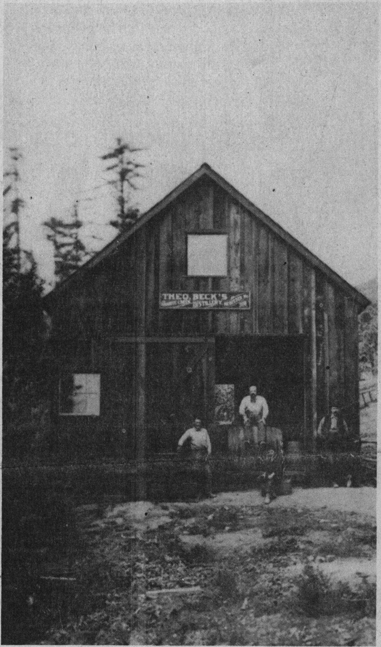
Theo Beck perched on a beer barrel for this view of his registered distillery on Granite Creek Road.
