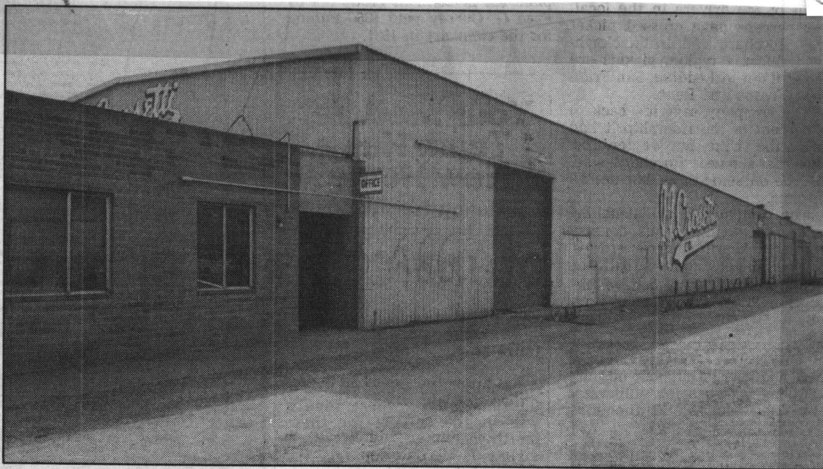
Familiar Crosetti plant will be turned into industrial complex
