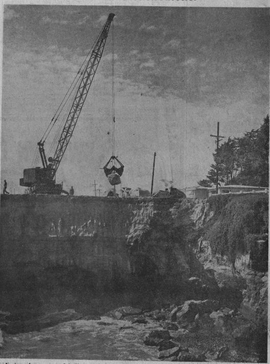
A towering crane daintily arches a five-ton boulder out over this cove at the foot of Columbia street as Granite Construction company begins work on the \$177,000 West Cliff erosion control program. The
