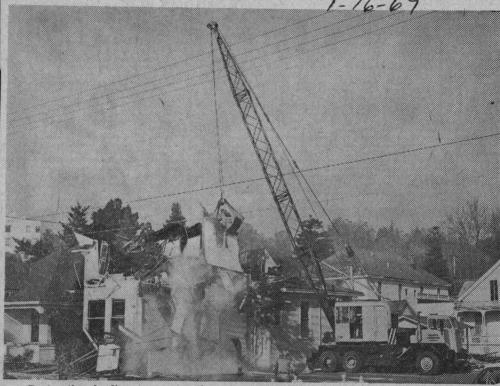
Destruction leading to construction of a two-story addition to the Santa Cruz city hall began today, as workmen for Granite Construction tore into four homes and other structures standing on the addition site. The
