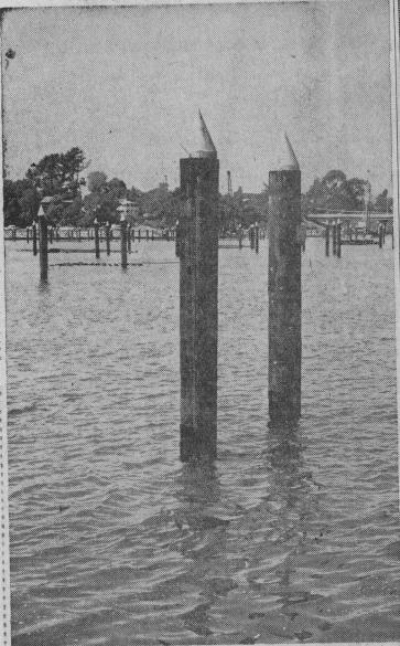
Seagulls, as picturesque as they may be, are not welcome at the new Santa Cruz harbor. To discourage the birds, each piling of the harbor is being equipped with a cone-like galvanized tin top. The sharp point is highly uncomfortable for gulls.
