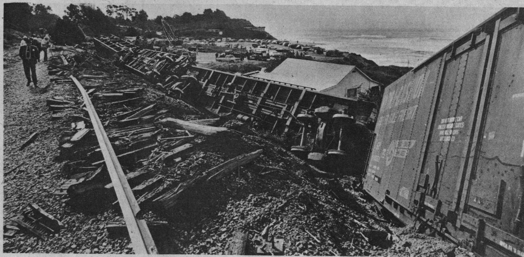
Repair crews had a big job ahead of them today, but Southern Pacific figures it can be done in two days.
