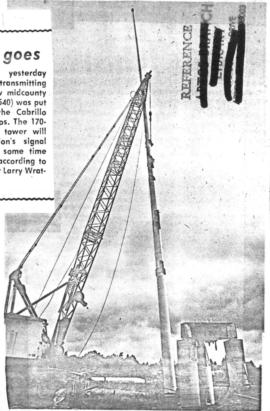
. . . lifted into a vertical position . . .
