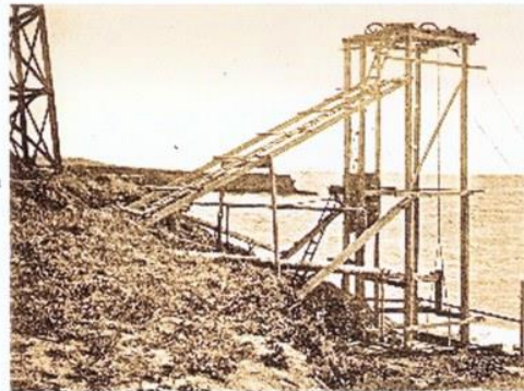
A view of the wave motor structure, looking south toward Stockton Avenue.
