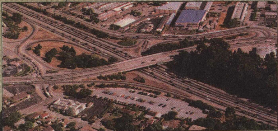
Soquel Avenue crossing.
