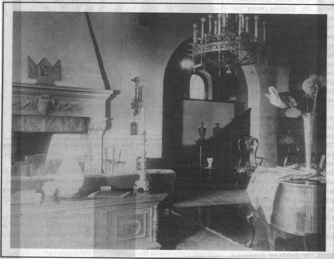
The fireplace, the windows and a portion of stairway are all that's left to identify this room.
