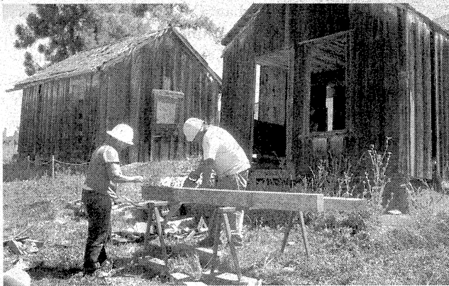
Left: Volunteers shore one of two remaining workers' cabins prior to performing work on its foundation. Above: In the mid-1800s, Santa Cruz County was the largest lime manufacturing area in California. Photos: Frank Perry
