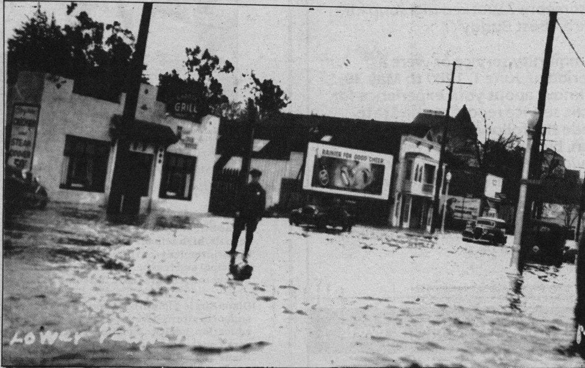
A Santa Cruz policeman directs traffic on lower Pacific Ave. during a flood in the early 1900s.
