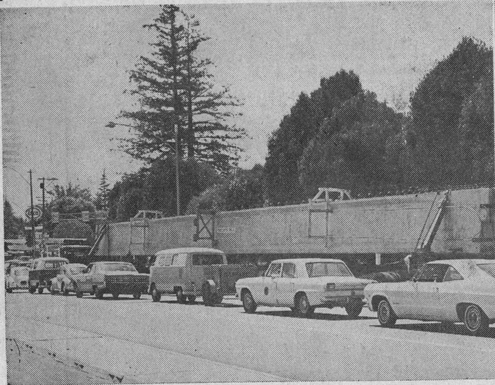
A massive moving job began Friday as the first of more than a score of prestressed concrete bridge girders arrived in Santa Cruz. Parked in the right lane of the Highway 1 freeway connection to Mission Street, it turned heads of motorists blocked up at the intersection. (Photo at left). For an idea of its size, count the number of cars next to
