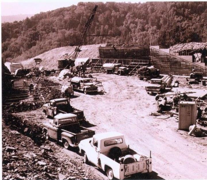
(Above) In 1960 crews began the construction of the Newell Creek Dam in the Santa Cruz Mountains. The body of water that formed behind the 195 feet high earthen dam was originally named the Newell Reservoir but then later changed to Loch Lomond.
