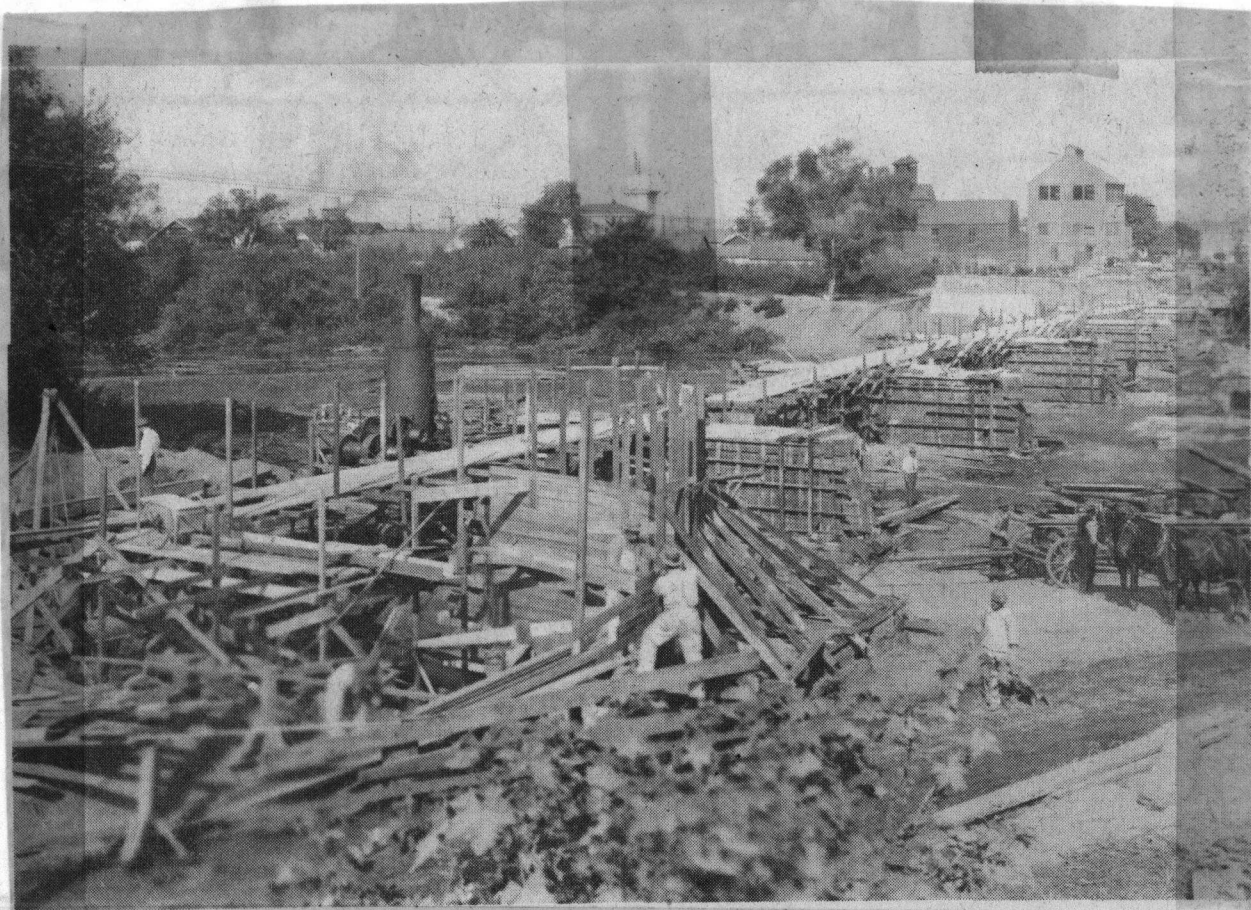
Workers put up the first concrete bridge, built in 1915.
