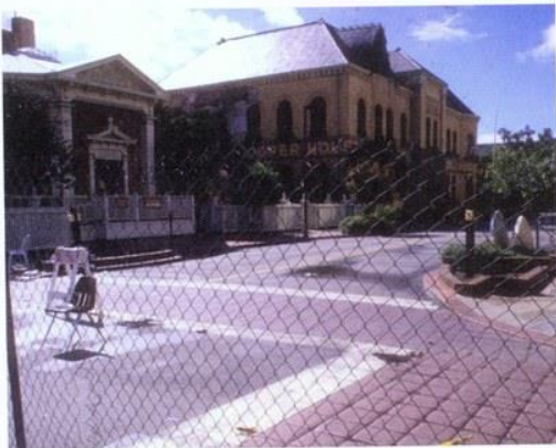
(Above) A deserted Cooper House stands behind one of the many cyclone fences that restricted access to Pacific Avenue after the Loma Prieta Earthquake.
