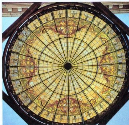
(Above) One of the two stained glass domes, originally installed in the First Presbyterian Church, were restored by John Forbes of Boony Doon Art Glass and installed in the Cooper House.
