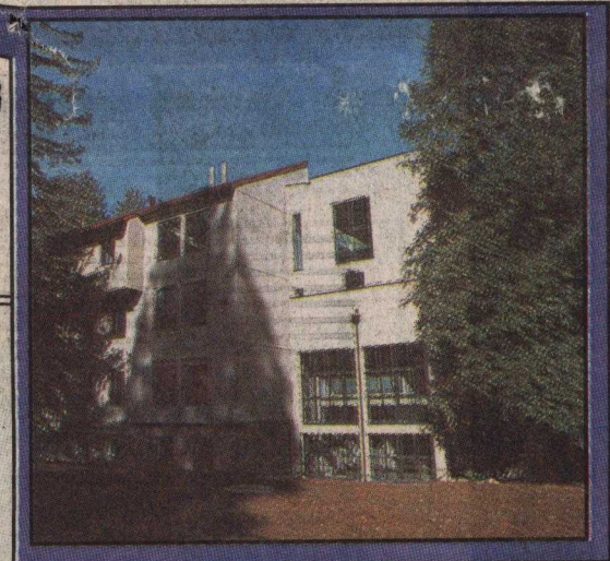
The new College Nine academic building is nearly complete.
