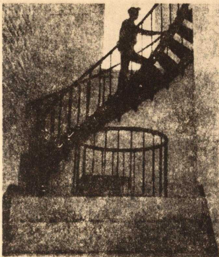
• At the bottom of the 133-step stairway, a railing surrounds the well into which weights from the ancient clock-works once descended
