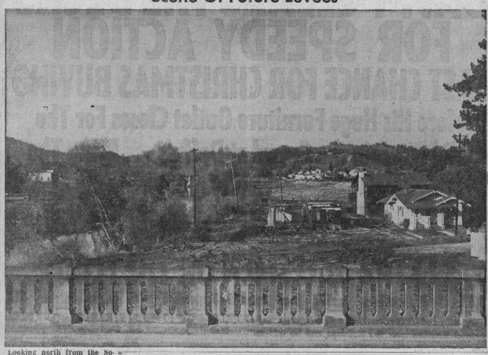
Looking north from the So-quel avenue bridge, the camera catches land clearance for lev-ees to be constructed next year along the San Lorenzo River flood control project. The semi-demolished house on the right and its adjacent neighbors will be cleared away soon for the project.
