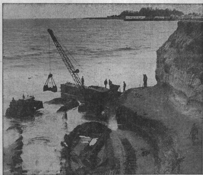
This is how the first section of the experimental groin going into the surf off Twin Lakes looked yesterday as army engineers filled the steel pontoons with sand ballast. The picture
