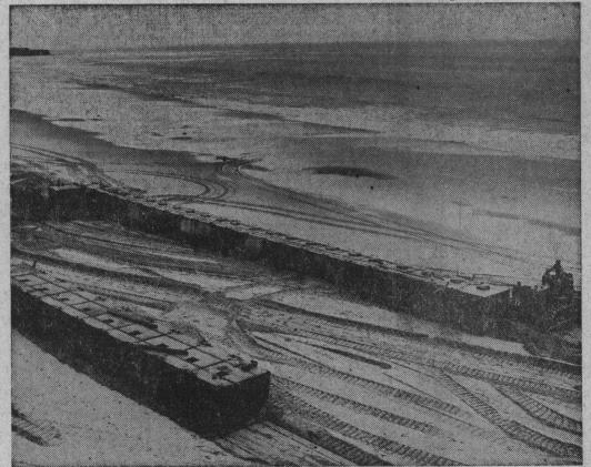
Army bulldozers are shown here pushing a groin section out of tide's way after this morning's attempt to place the experimental structure off Twin Lakes beach ended in defeat. Section in foreground
