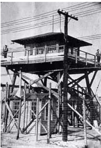
Watch Tower, Poston, Arizona, 1942
